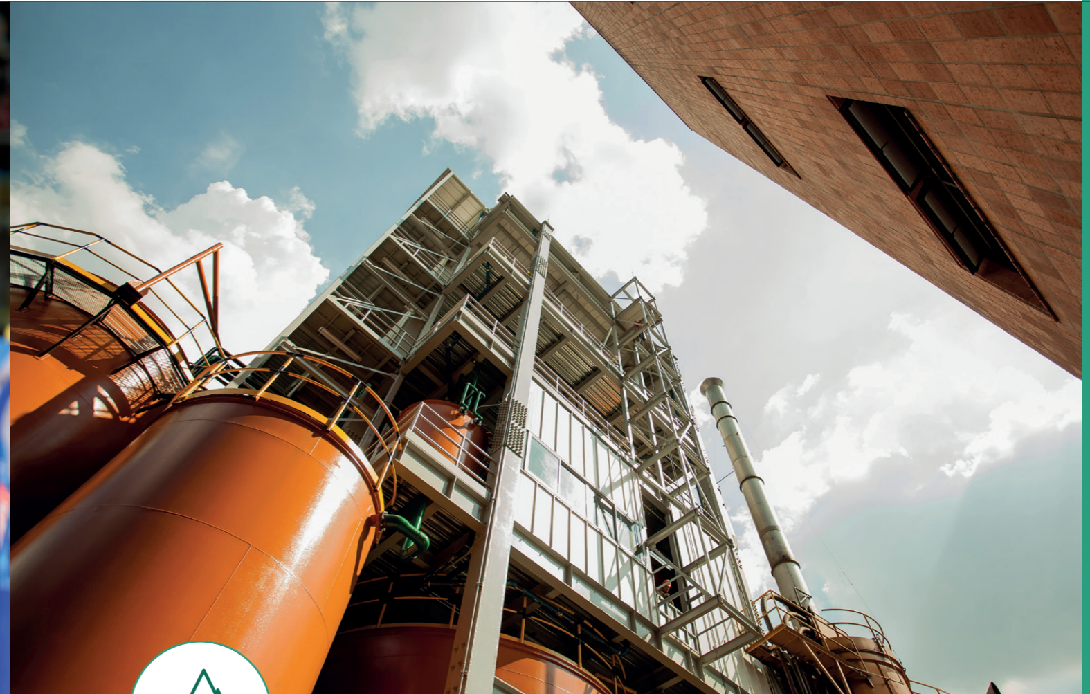
»»» Wastewater treatment plant at the Coffee Business facilities in Medellín, Colombia.
